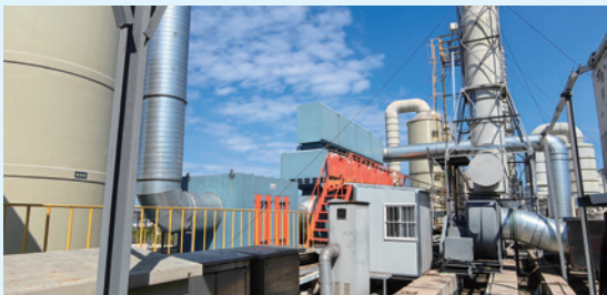
Exhaust Gas RCO Treatment Upgrade Project
